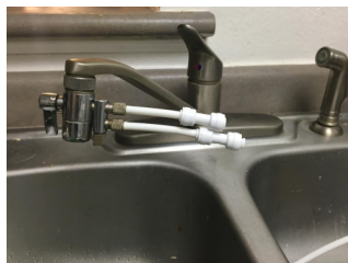
On picture - dual diverter. Single diverter can be connected/disconnected the same way
