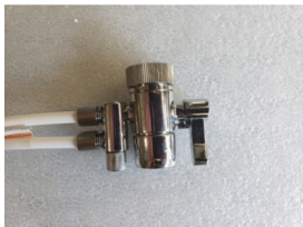
5. Screw the nuts onto the inserts by hand, then tighten with pliers.
