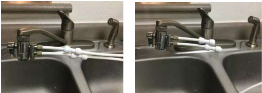
The picture shows a dual diverter. A single diverter works the same way.
